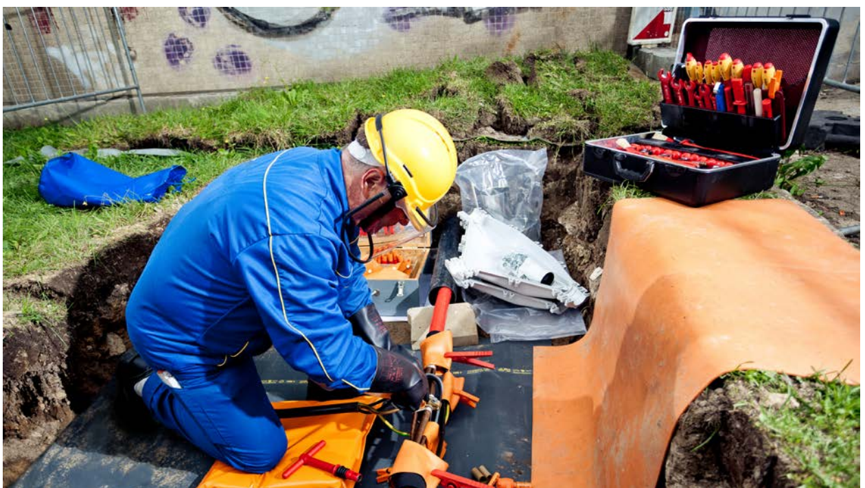
Abb. 21 Muffenmontage: k_r = 1,9
